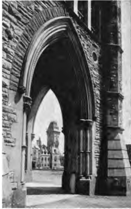
MAIN ENTRANCE, CENTRAL BLOCK.
